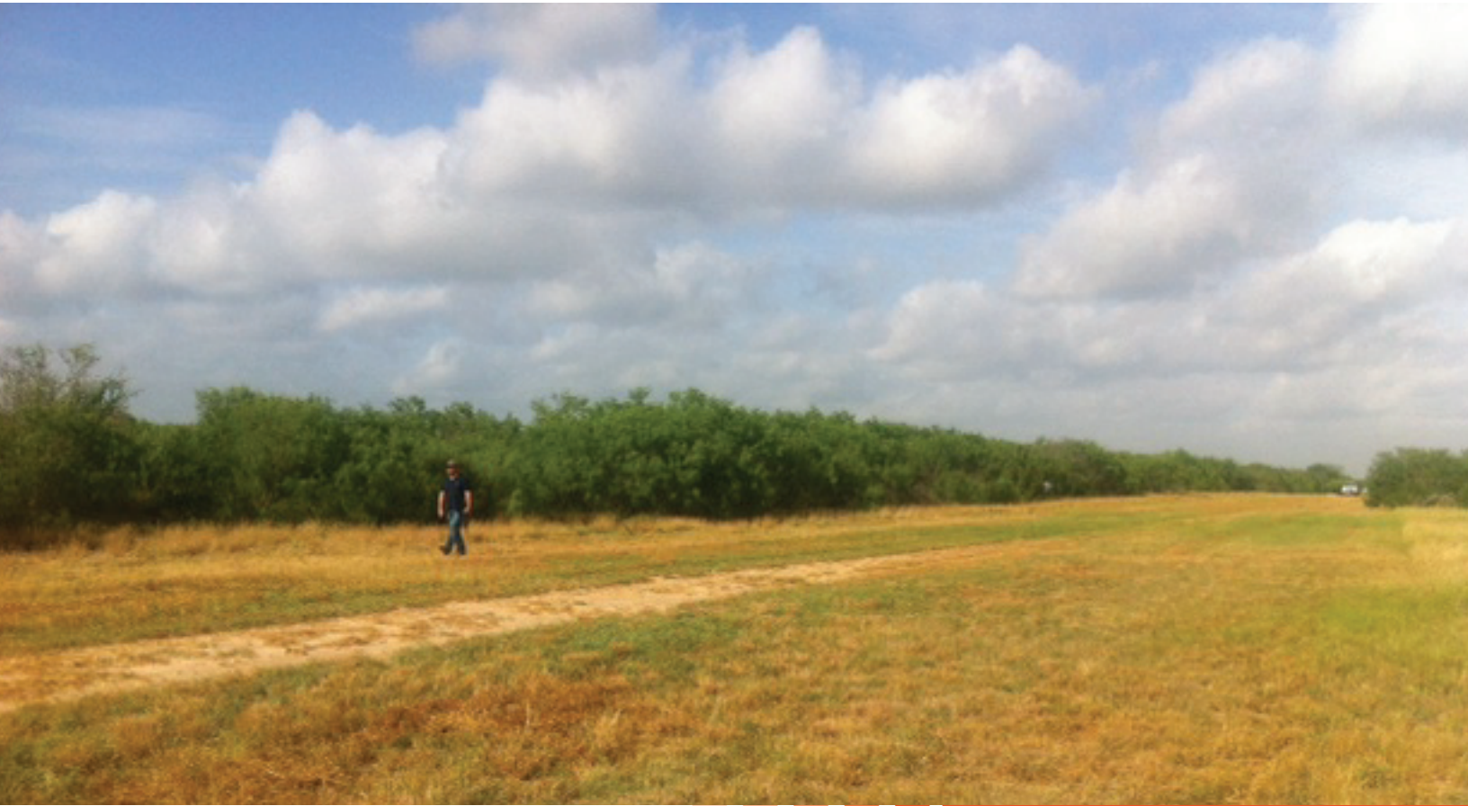
A view of the pipeline location and service road.
